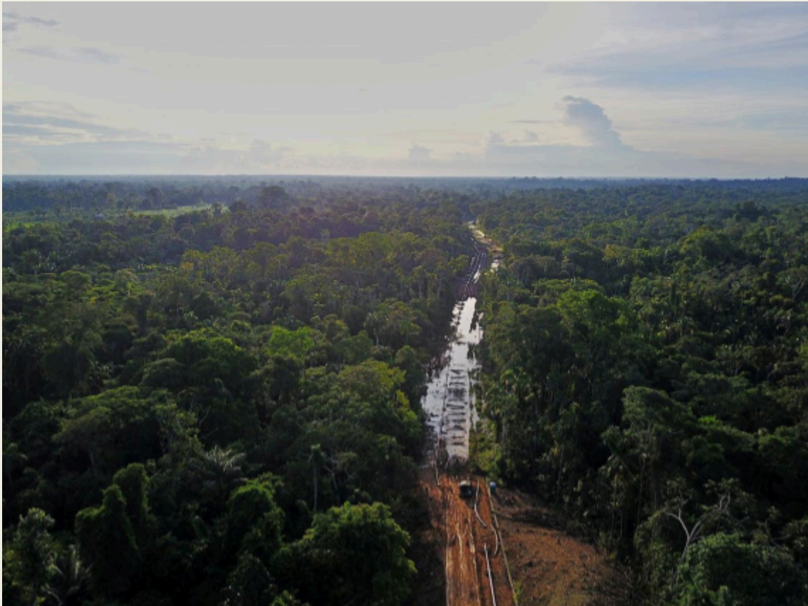
The oil industry has been the main driver of deforestation in the Ecuadorian Amazon for decades. Roads and oil pipelines built to access oil facilities—such as this one, near the ancestral lands of the Siona people, built by the Chinese oil giant Andes Petroleum—often strike the rainforest's integrity first, followed by settlement. Amazon Frontlines created this map of oil ponds in October 2017. Photo: Mitch Anderson / Amazon Frontlines.
